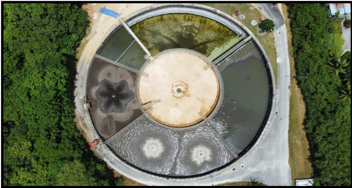
The current aerial photo of the main circular clarifier. PEP is working in the centre part.
