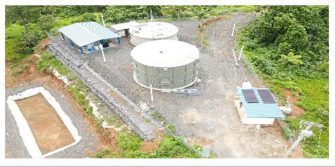
Figure 2. Aerial View of Vunidawa WTP
