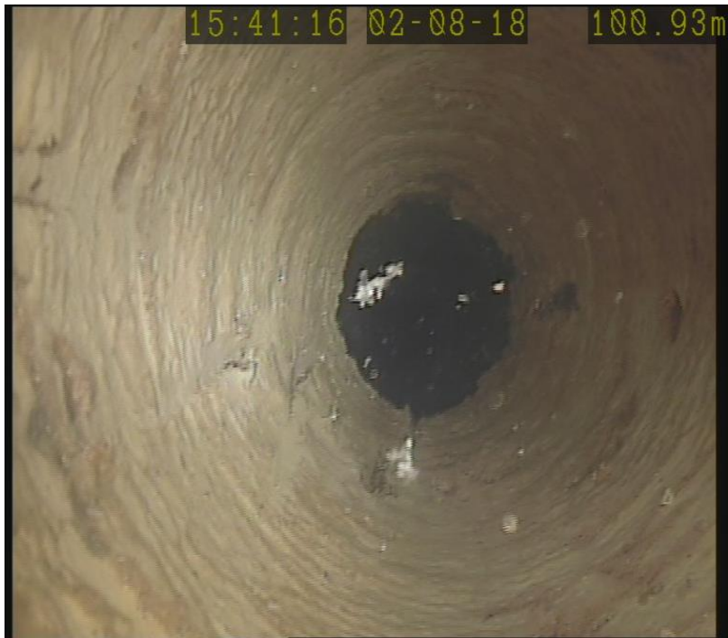
Calcite Deposition
